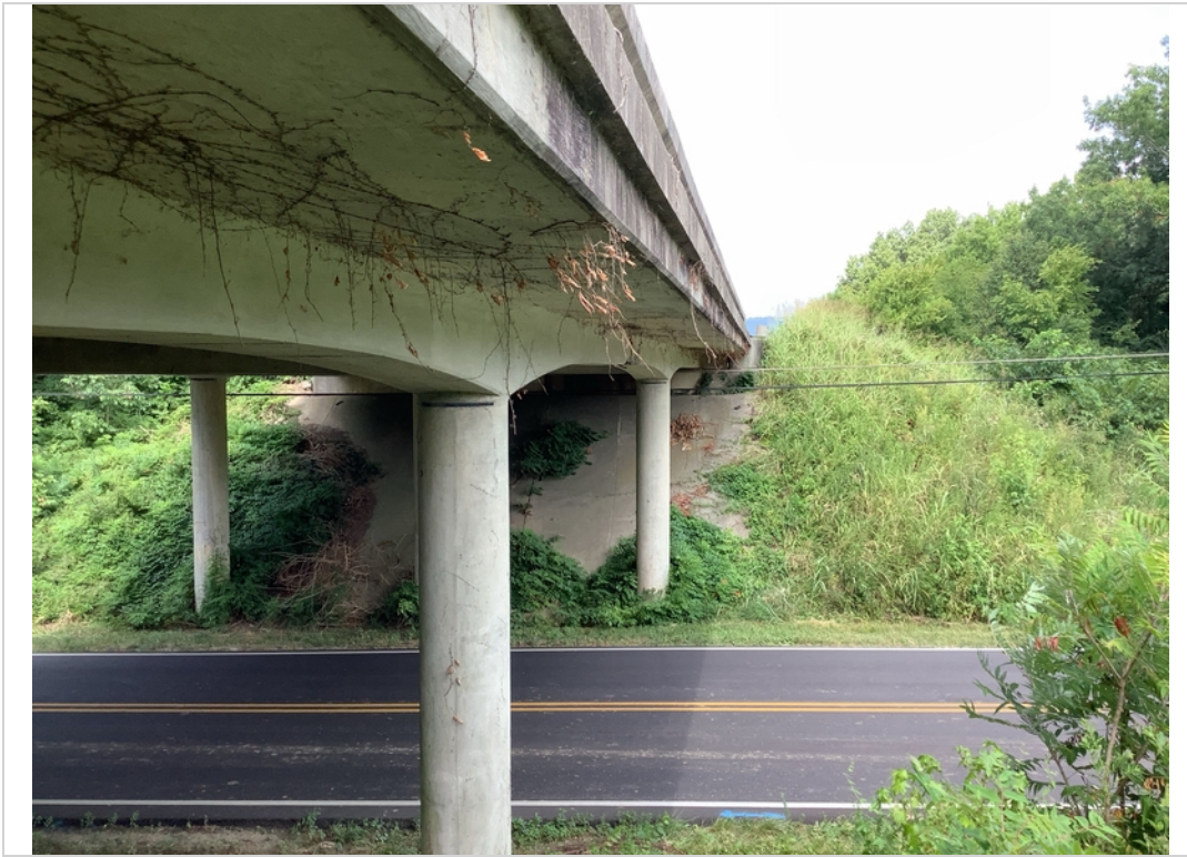
Left side view of structure
