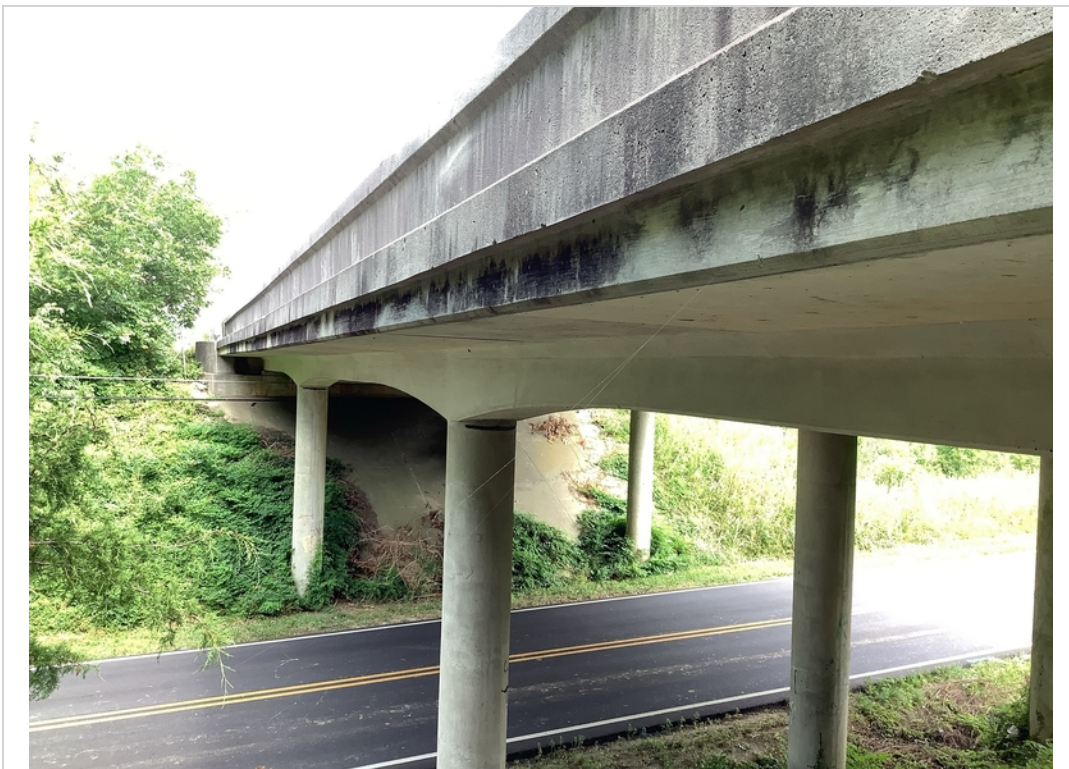
Right side view of structure
