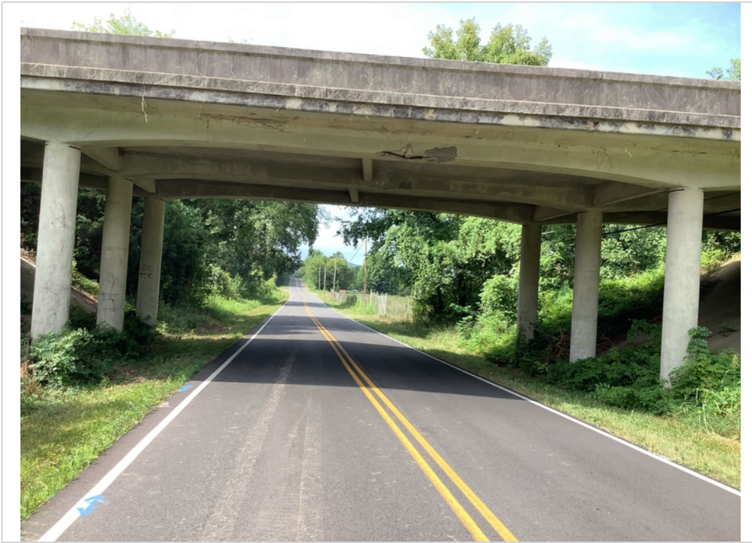
Underclearance looking ahead on underpass route
