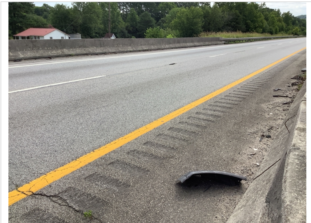
Top of deck
